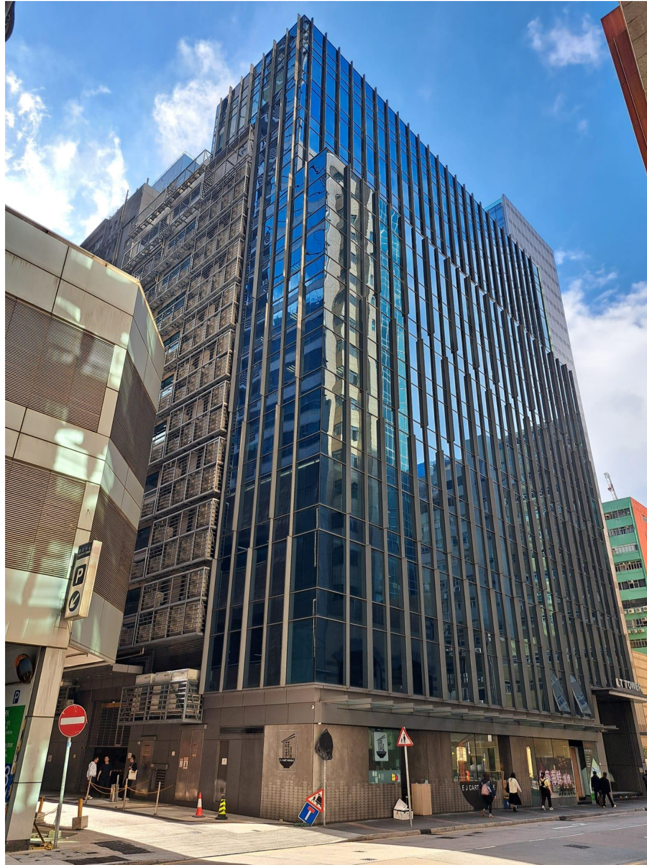
Photo 2 - Northern facade of the building
